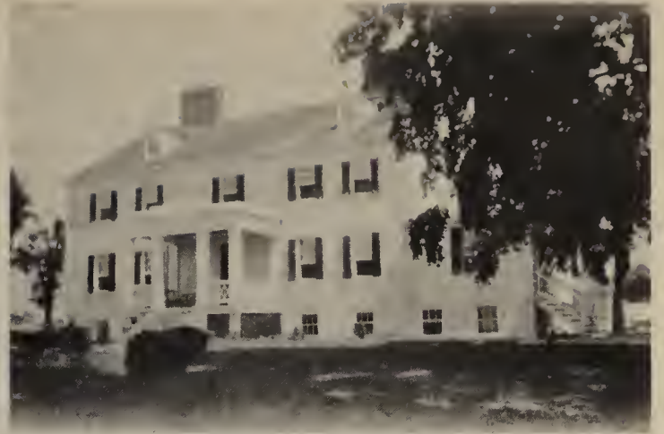
OAK HALL, HOWARD COUNTY, MARYLAND
