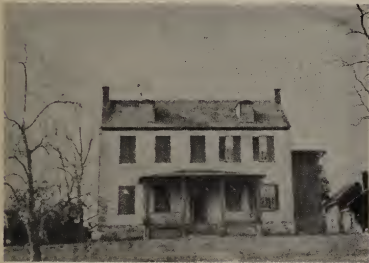
FONT HILL, HOWARD COUNTY, MARYLAND
